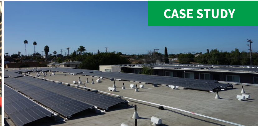
The Allison Apartments Rooftop Solar PV
